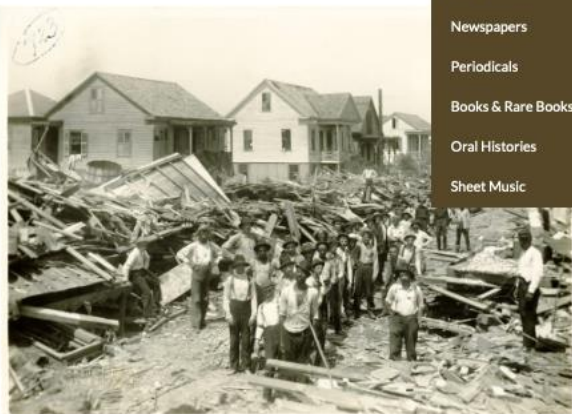
Posed group of workers during 1900 Storm recovery. G. 1771.7 FF3 12. Galveston Photographic
